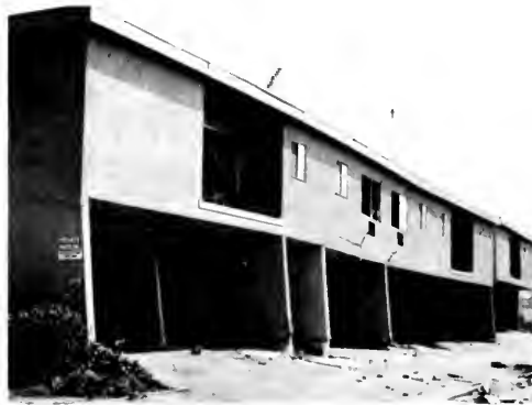
Photo 4. This apartment building, an Foothill Boulevard near Maclay Avenue, was damaged by both vertical ( 21'' \pm ) and horizontal ( 12'' \pm ) motion. Carport type of garage under second story dwelling is very susceptible to earthquake damage. Photo courtesy of City of Los Angeles Department of Building and Safety.
